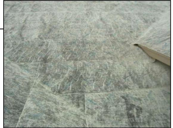
the installation of new shingles. When asphalt-saturated felt is used, the UV draws the oils right out of it and the underlayment is already deteriorating before shingle installation begins.
