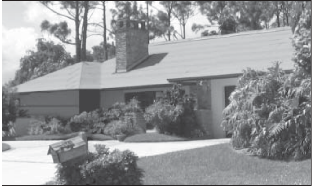
LeakBarrier Fast90 from Tarco survived the fury of Wilma when she passed through the Palm Beach area. Intended for use as a tile underlayment, Fast90 was serving as a primary roof for these residential homes because of delays in the delivery of tiles. (Photographs courtesy of Always Roofing, Lake Worth, Florida.)
