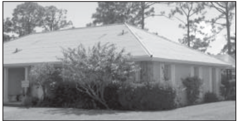
LeakBarrier Fast90 from Tarco survived the fury of Wilma when she passed through the Palm Beach area. Intended for use as a tile underlayment, Fast90 was serving as a primary roof for these residential homes because of delays in the delivery of tiles. (Photographs courtesy of Always Roofing, Lake Worth, Florida.)
