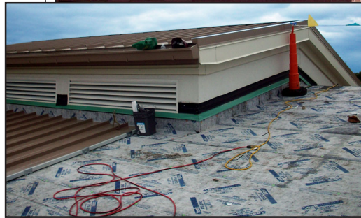
Tarco LeakBarrier® PS200 HT self-adhering underlayment provides a watertight secondary water barrier beneath metal roofing on schools in the Manteno School District.
