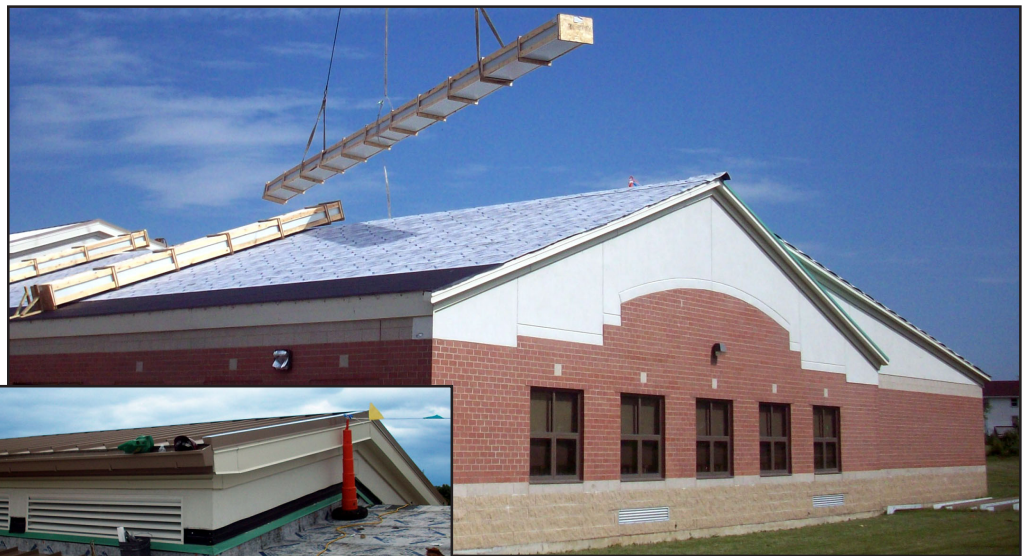
Tarco LeakBarrier® PS200 HT self-adhering underlayment provides a watertight secondary water barrier beneath metal roofing on schools in the Manteno School District.
