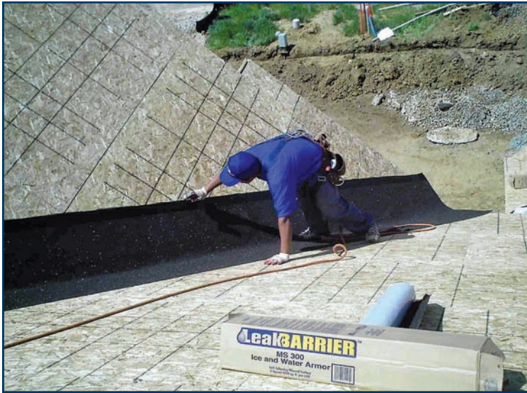
Figure 2 – LeakBarrier® MS300 Ice and Water Armor is highly effective in critical roofing areas such as valleys, ridges, coping joints, chimneys, vents, dormers, skylights, and low-slope sections.
