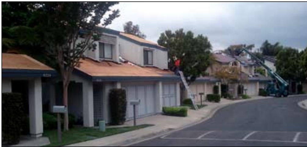
*The roofing systems are installed on four to six buildings at any given time. Here are three units at various stages of production.*
