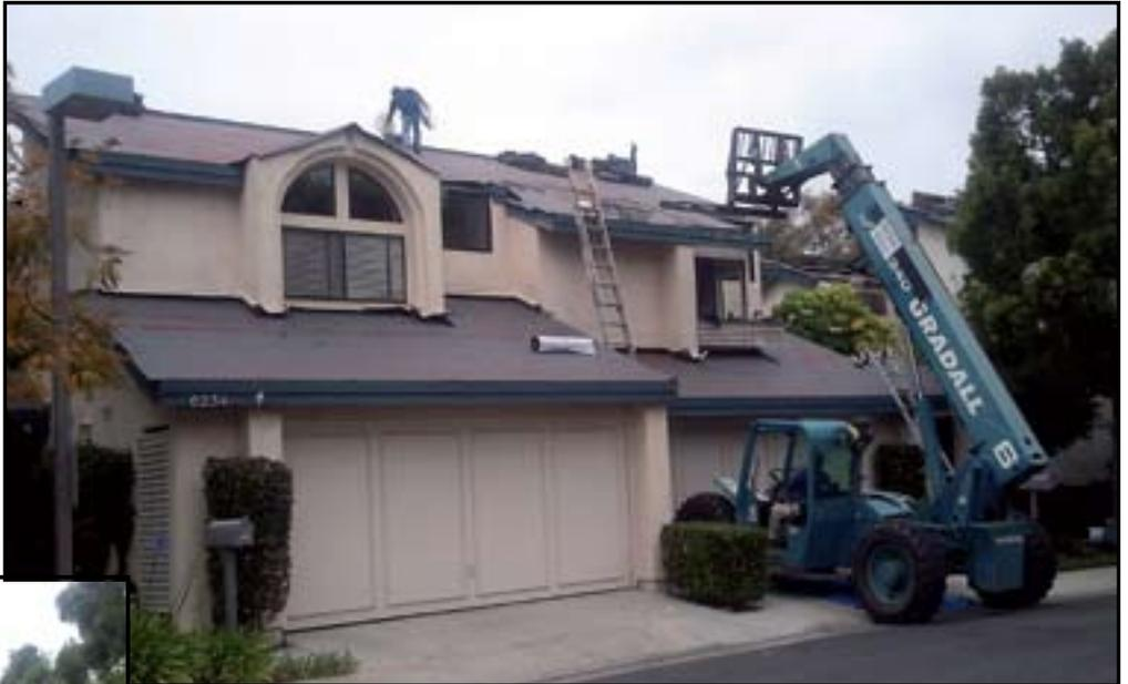
*Using EasyLay as a tile roof underlayment, a work force of 10 to 14 roofers reroofed these multiple unit buildings at a pace of about 12 to 16 buildings per month. The total number of units was 106.*
