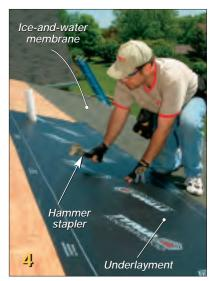
Fasten the underlayment to the decking. We used staples, but if the underlayment will be exposed to the elements for a lengthy period of time, use plastic-cap roofing nails.
