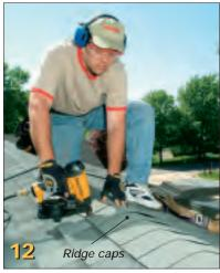
Special ridge shingles are used to cover the crown of the roof. If your brand doesn't offer ready-to-install ridge shingles, you can make your own from the tabs cut off of full shingles.
