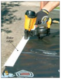
Apply drip edge to the roof rakes to enhance the performance of the underlayment and achieve a longerlasting roof.
