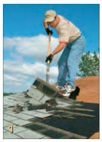
Use a roofing shovel to strip off the old shingles and underlayment. Be sure to remove all nails and staples.
