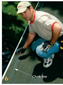
Snap a line to indicate the placement of the starter shingles. Use red chalk because it withstands foot traffic and won't rub off as easily as blue chalk.
