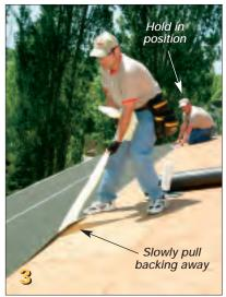
Carefully position ice-and-water membrane, and have a helper hold it in place. Gently pull away the backing to expose the adhesive, and press down to adhere the membrane.
