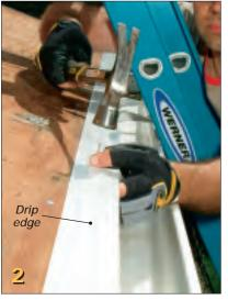
Use 1-1/4-in. roofing nails to attach new drip edge to the eaves. Set nails every 16 in., and overlap sections of drip edge to ensure consistent protection.
