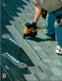
Fasten subsequent courses of shingles in a staggered pattern. Follow the manufacturer's instructions for the recommended offset.
