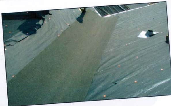
MODIFIED BITUMEN BEING USED IN A ROOF VALLEY ON A RESIDENTIAL PROJECT.
