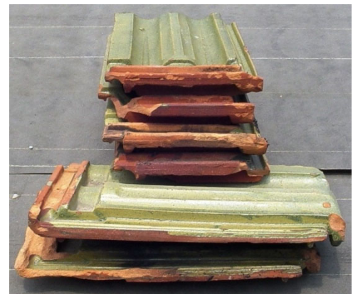
Side View - Staged Tiles (Slope ↓)
